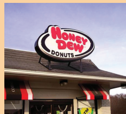
Roof Mounted Signs
