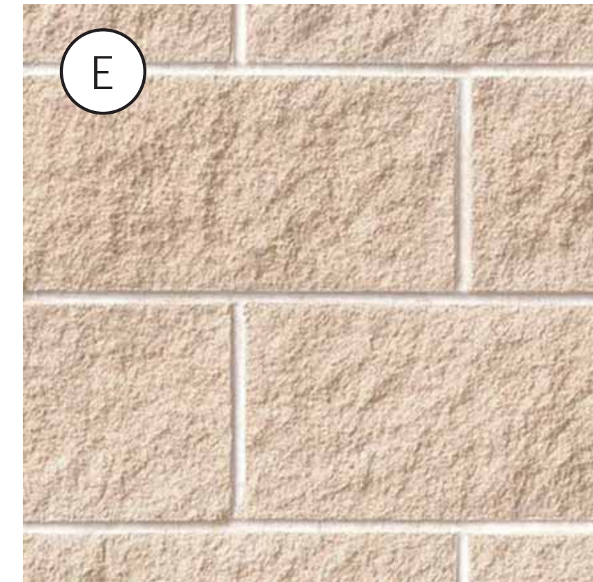
E CONCRETE MASONRY UNIT BLOCK WALL
