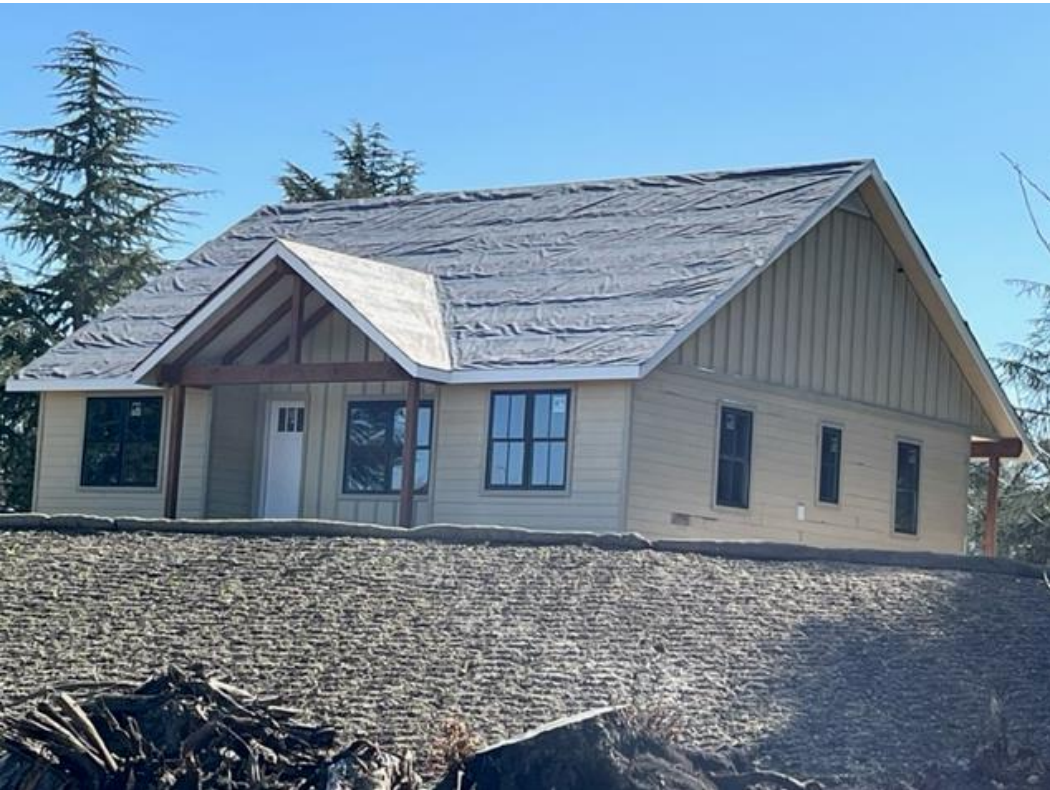
New house under construction
