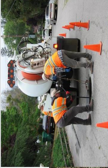
FOG build-up in sewer pipes (shown below) is costly to clean requiring local Public Works staff to go to the site & remove
