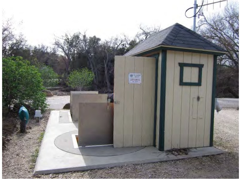
Figure 6-8: Lift Station No. 9 is in good condition.
