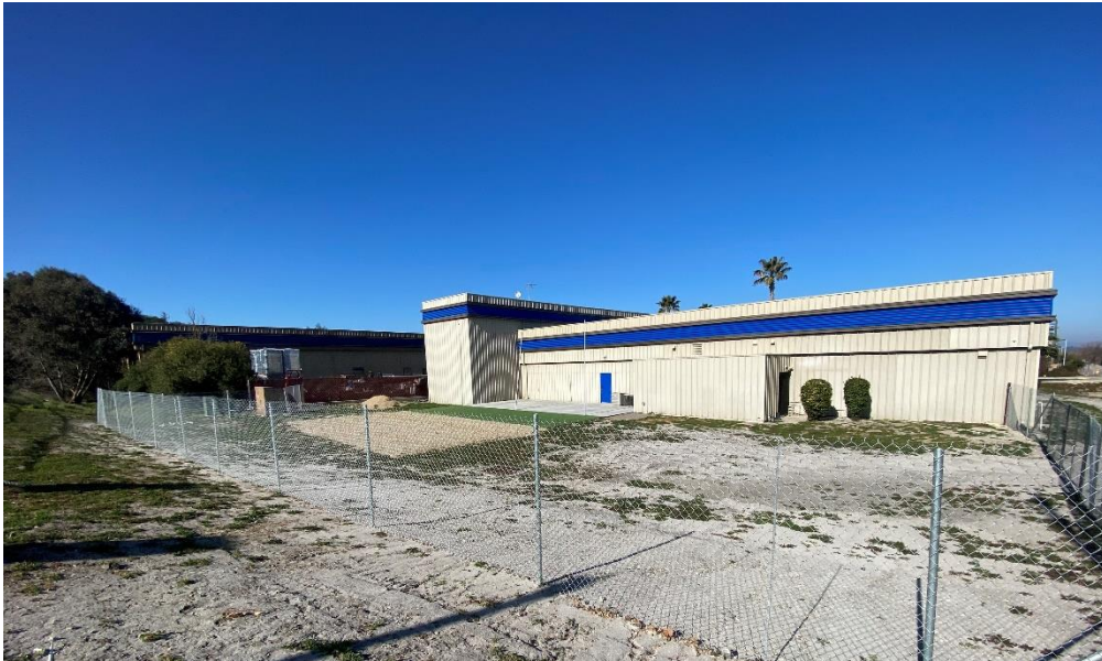
Sides of Existing Building
