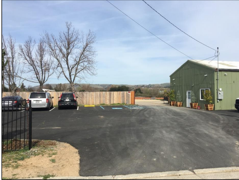
Existing Frontage and Access from Via
