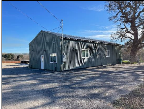
Existing Office Building
