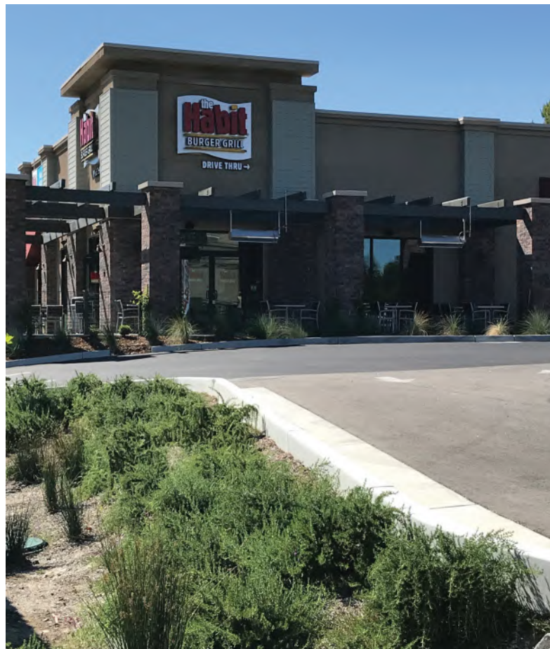
Example of new commercial project with landscaped water-quality-treatment swale in front.
